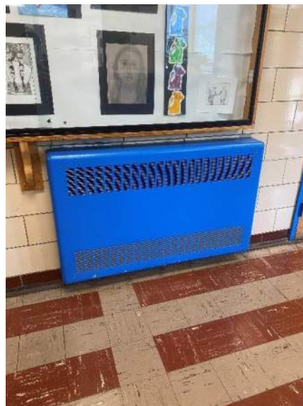
Typical hydronic radiator
