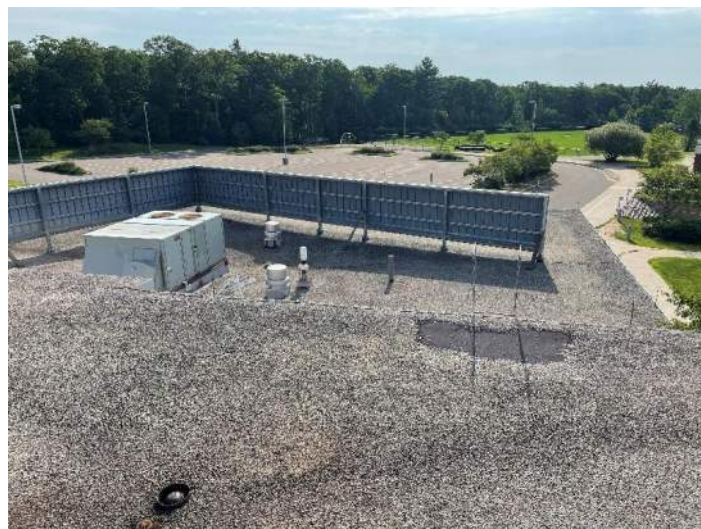
D.1.10: Exterior – Roof – Gravel Built-Up – Central Wing
