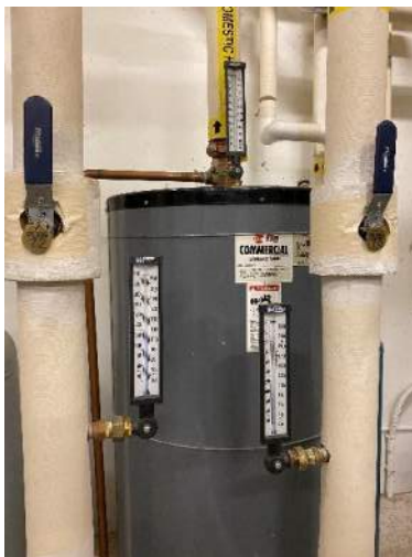
D.2.1: Rheem Domestic Hot Water Storage Tank
