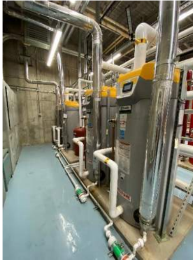
D.2.1: Four Domestic Water Heaters Serving the High School
