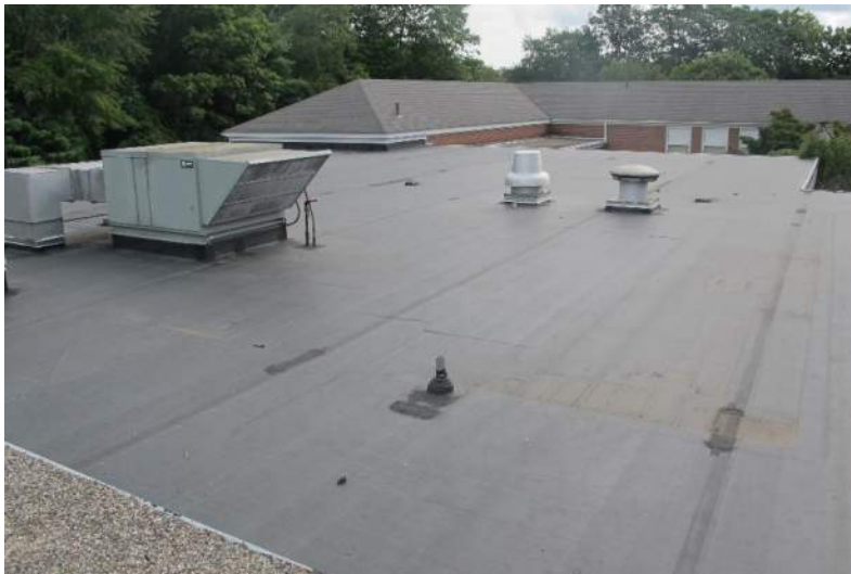
D.1.12: Roof – EPDM Membrane – Vintage 2
