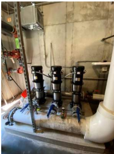
D.2.8: Domestic Water Pumps within Pump Vault
