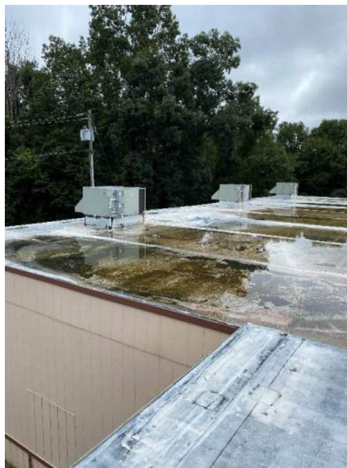
Packaged Roof Top Units
