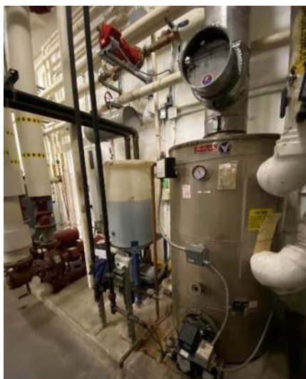
D.2.2: Aldrich Oil Fired Domestic Hot Water Tank
