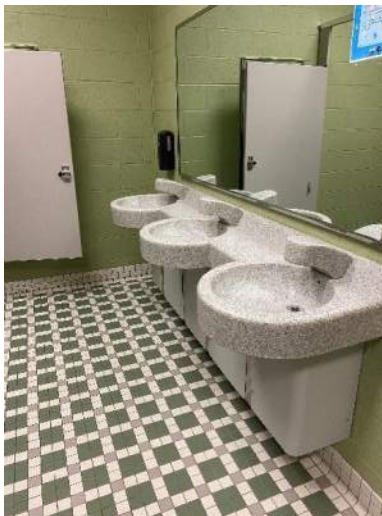
D.2.7: Sensor Operated Plumbing Fixtures
