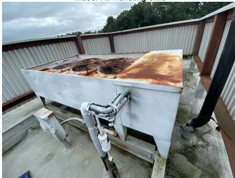
Associated outdoor condensing unit
