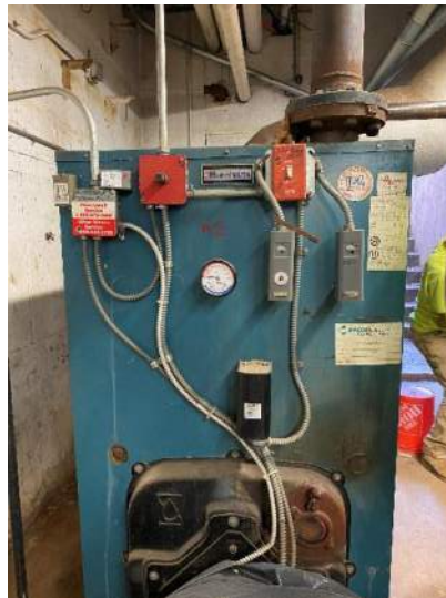
D.2.3: 1989 Boiler Room Hot Water Boilers
