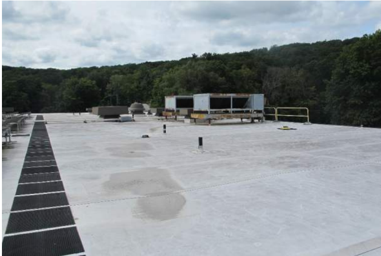
D.1.12: HKHS Roof – EPDM Membrane
