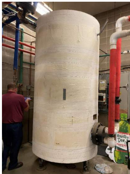
Hot Water Storage Tank
