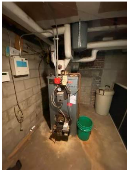
D.2.10: White House Hot Water Boiler
