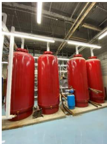
D.2.4: Four Hot Water Expansion Tanks
