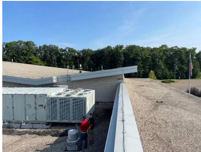
D.1.9: Exterior – Roof – Gravel Built-Up – North Wing
