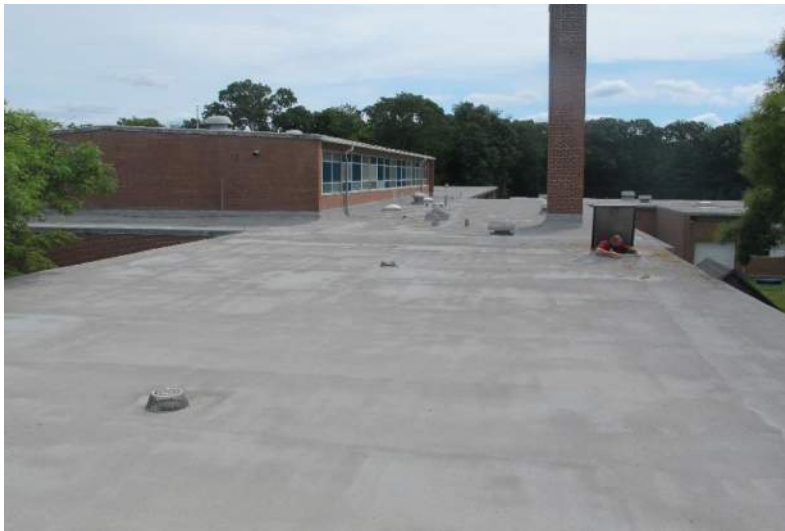
D.1.39: Central Office – Roof – Spray Polyurethane
