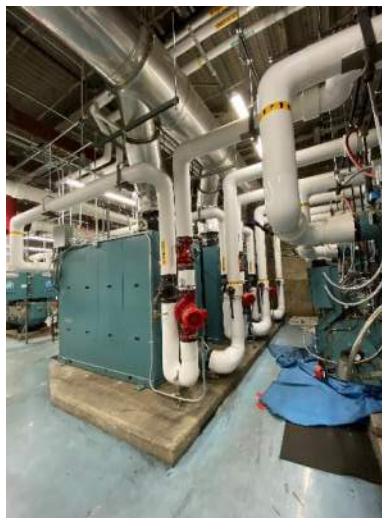
D.2.2: Six Hot Water Boilers
