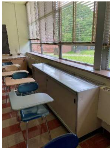
D.2.12: Central Office Building Unit Ventilator
