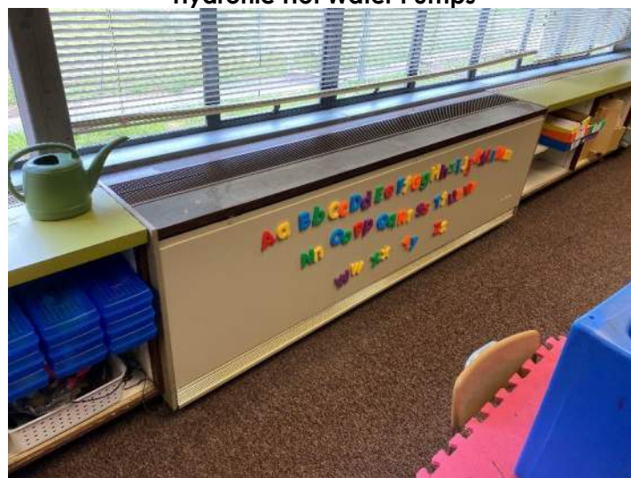
Typical Classroom Unit Ventilator
