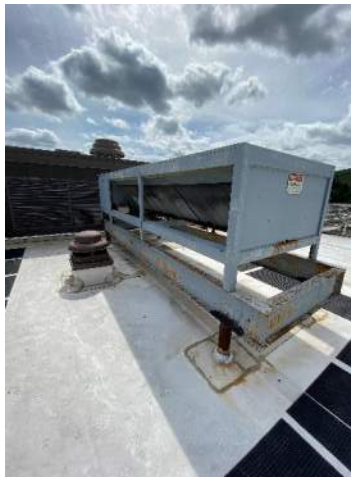
D.2.7: Condenser Unit Located Outside on the Roof
