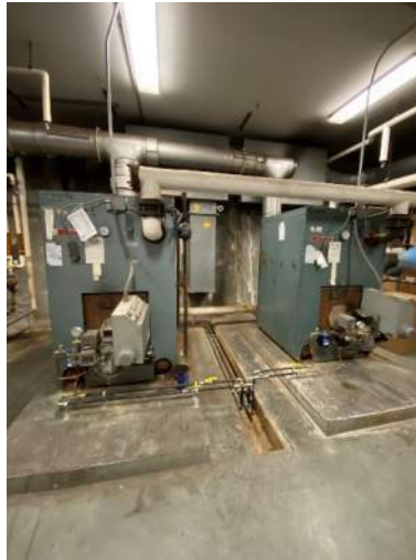
D.2.3: 1989 Boiler Room Hot Water Boilers
