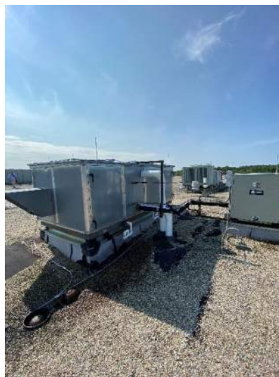
D.2.6: Trane Rooftop Unit with Air-Cooled Condensing Unit
