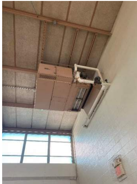
Typical Unit Ventilator serving gym
