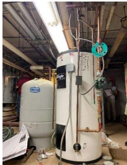
D.2.2: 1948 Mechanical Room Domestic Water Heater
