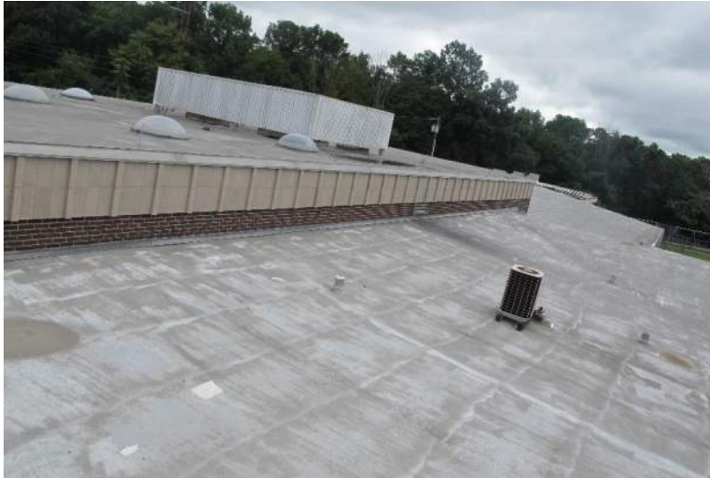
D.1.11: Roof – Spray Polyurethane – Vintage 1
