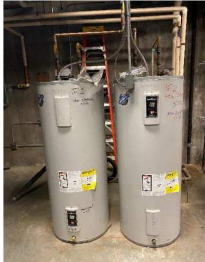
D.2.1: 1989 Boiler Room Domestic Water Heaters
