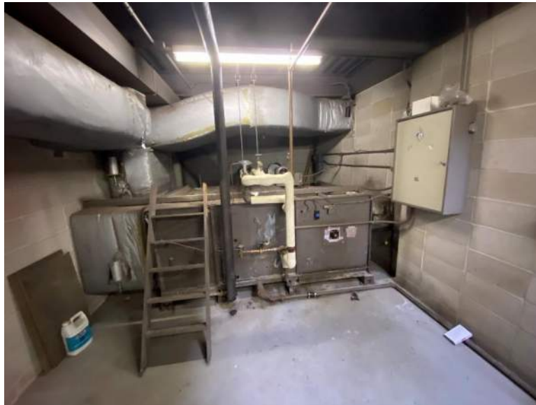
Indoor Air Handling Units
