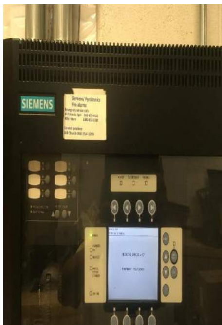
EXISTING FIRE ALARM CONTROL PANEL
