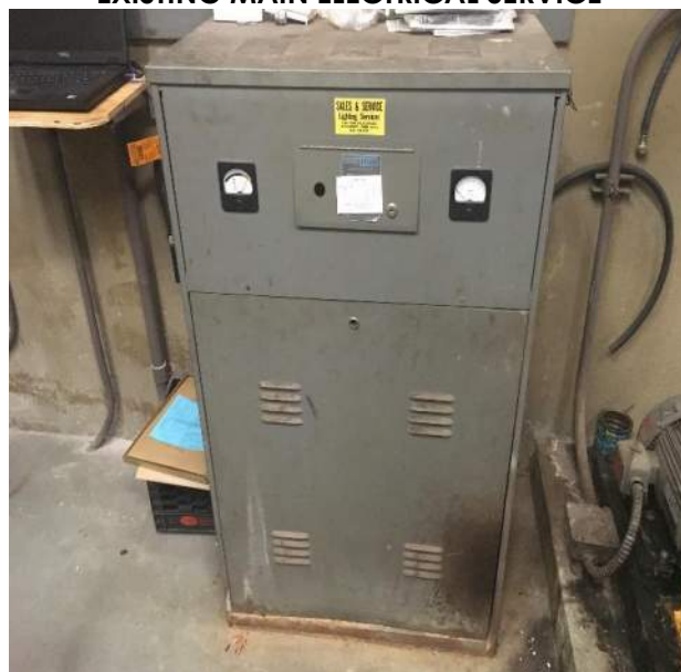
EXISTING EMERGECENY LIGHTING BATTERY UNIT
