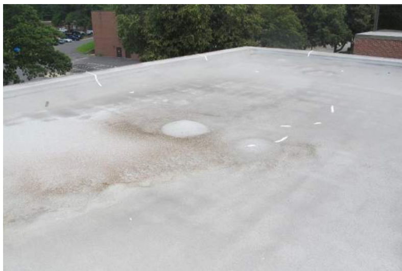
D.1.11: HKHS Roof – Spray Polyurethane
