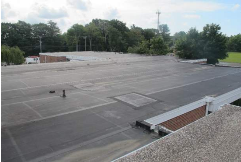
D.1.13: Roof – EPDM Membrane – Vintage 3
