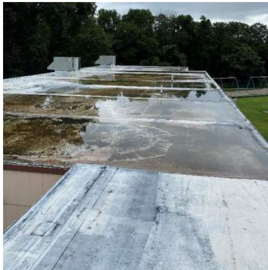
D.1.12: Roof – EPDM Membrane – Vintage 2 Modular Units
