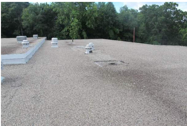
D.1.14: Roof – Gravel Built-Up – Vintage 4
