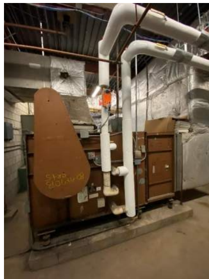
D.2.6: Air Handling Unit Serving the Pool Room
